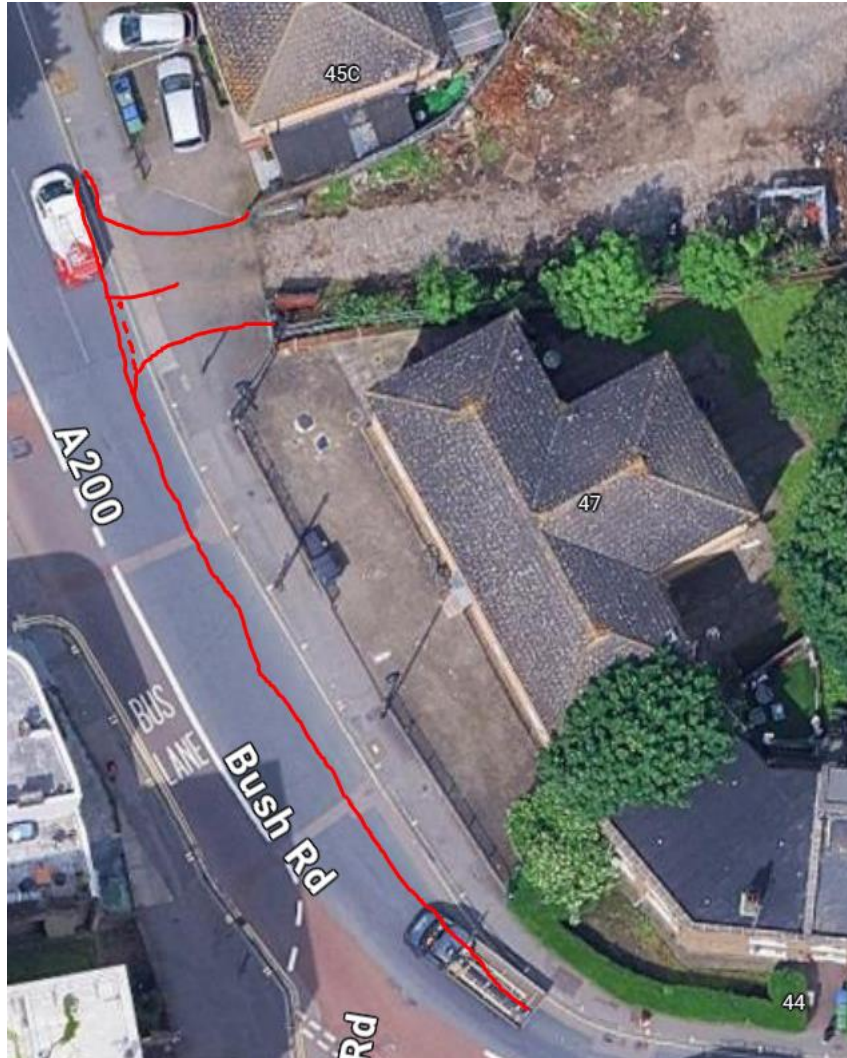
Bend along Bush Road towards Development site
