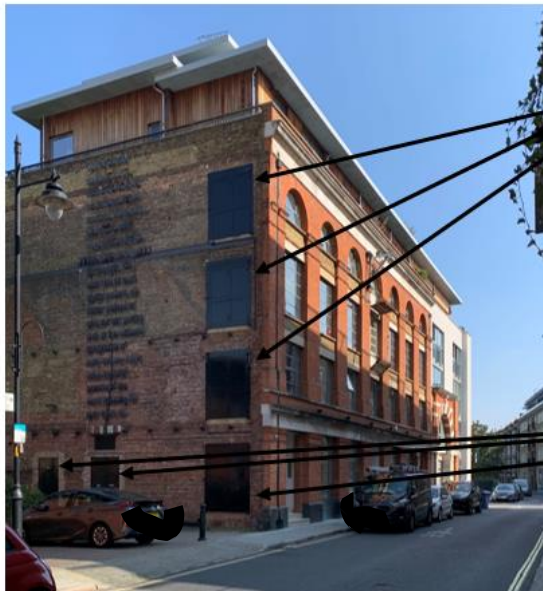
Image – Loading bay doors
