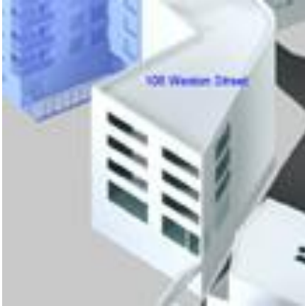
Image – north elevation of 106 Weston Street
